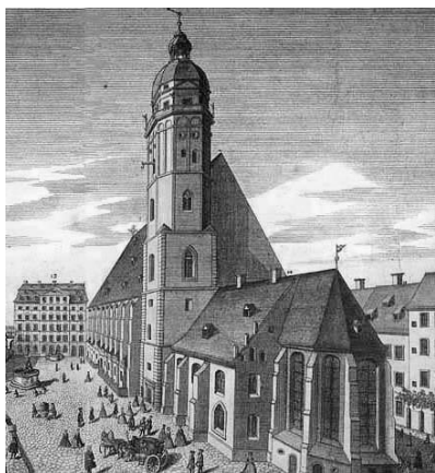
Engraving (1735) of the Thomaskirche and Thomasschule (distant, left)
